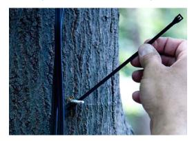
Step 2. Thread cable tie through eyebolt and around wire(s).
