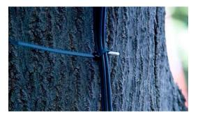
Step 3. Close cable tie loosely to allow for movement of cable through tie. Trim excess cable tie.
