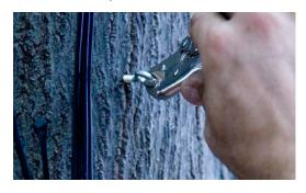
Step 1. Predrill hole then secure stainless steel screw eyebolt. Leave about 1" thread exposed.
