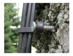
This method has the advantage of allowing the installer to back off the screw as the bark expands. The eyebolt method requires cutting and changing the cable tie as the tree grows.
